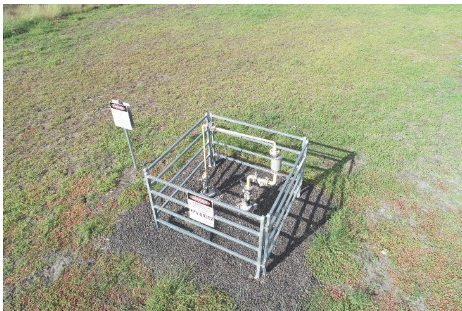
Figure 10 High point vent (HPV)
