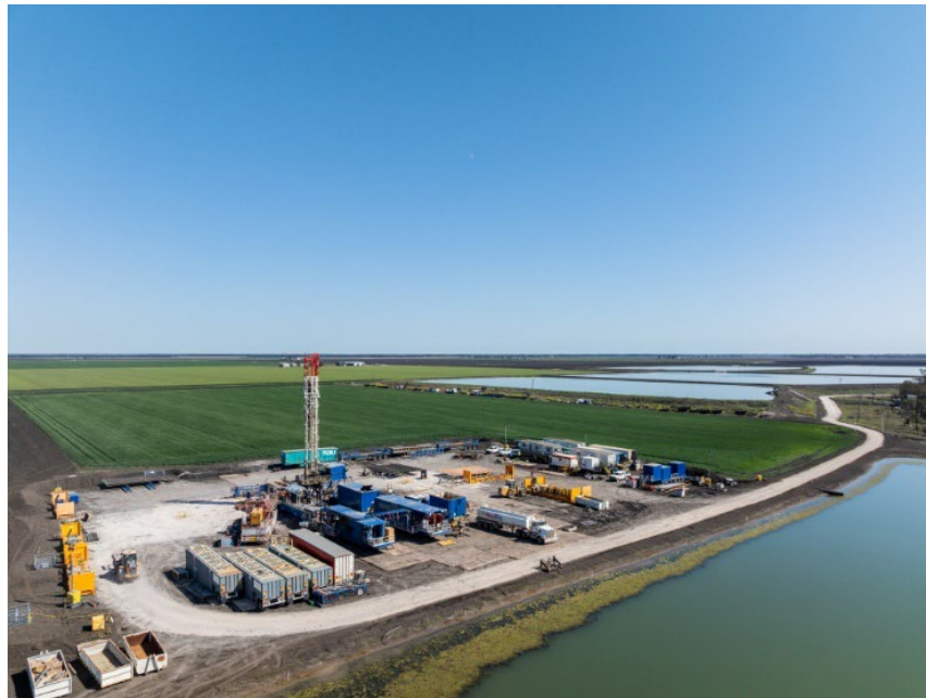
Figure 7 Typical Drilling Rig
