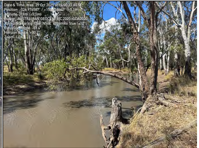
Plate 13: Facing upstream towards crossing on Sixteen Mile Creek (on lot plan 2RP82810)
