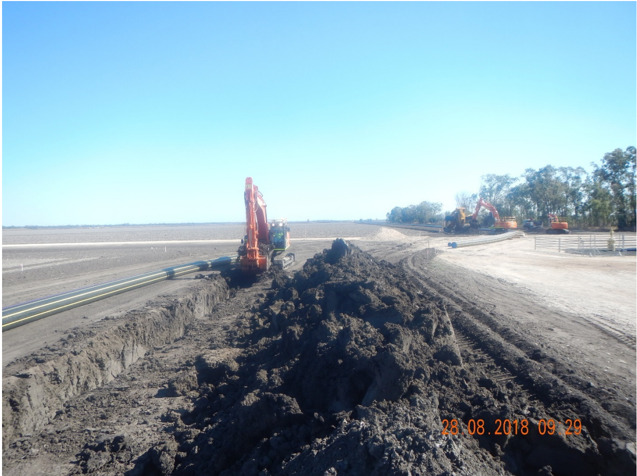
Plate 3-2 – Image of pipeline being installed by trench method
