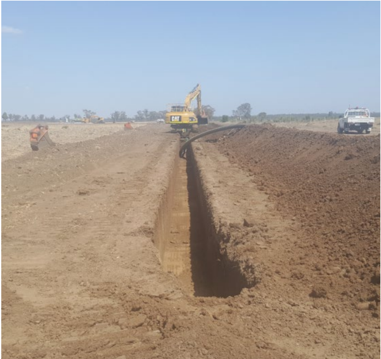
Plate 3-1 – Image of pipeline being installed by trench method
