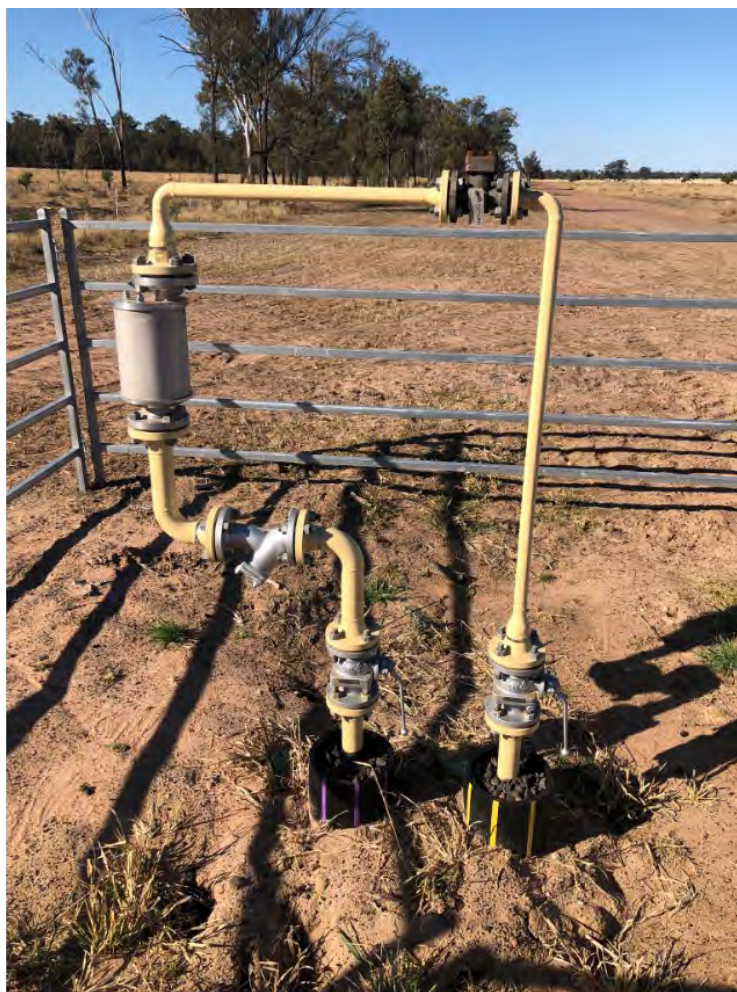
Plate 4-9 -- Image of a High Point Vent
