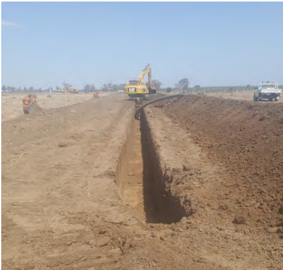
Plate 4-10 – Image of pipeline being installed by trench method
