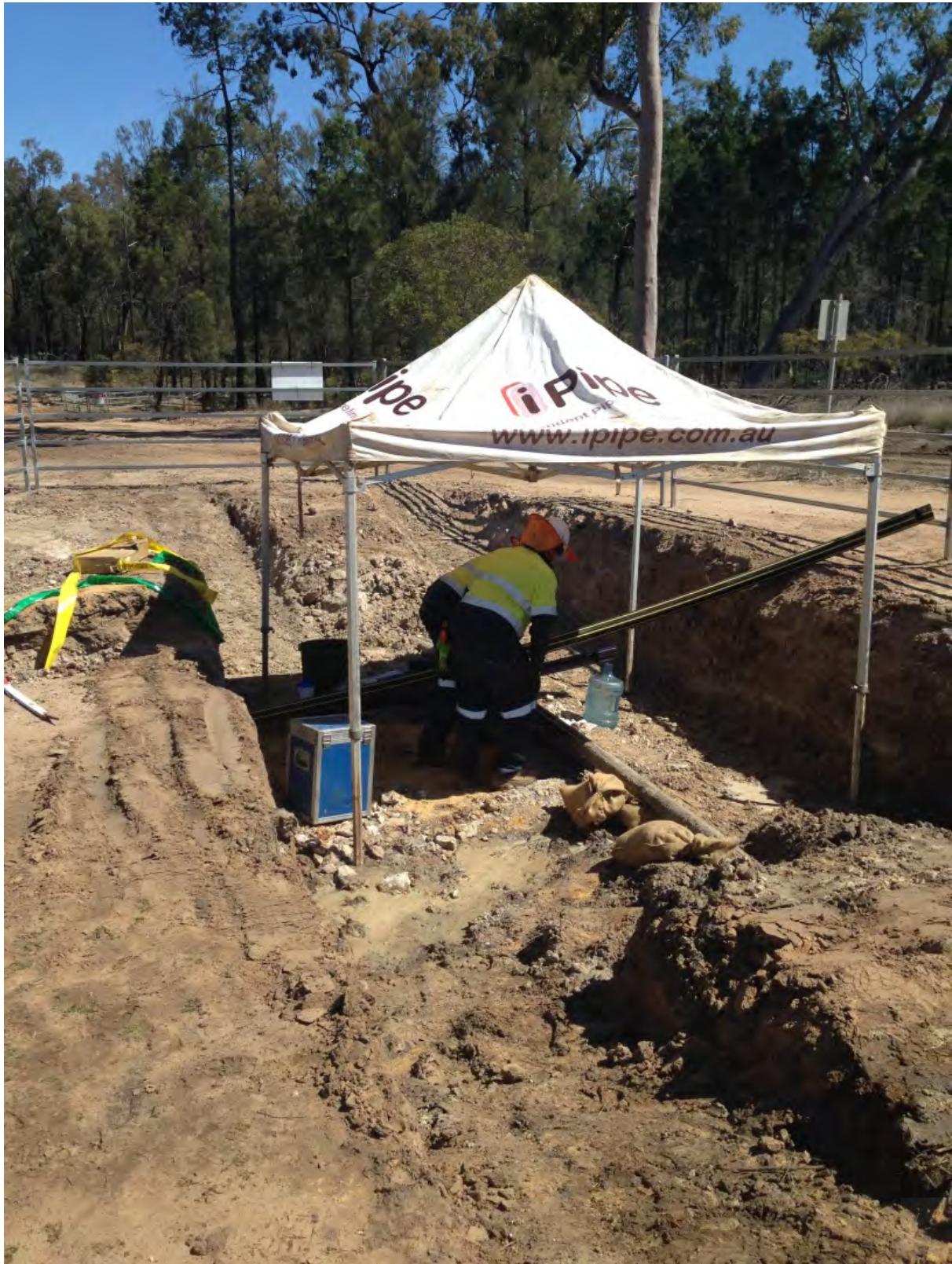
Plate 4-7 – HDPE gathering being installed
