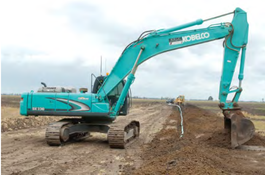
Plate 4-11 – Backfilling pipeline trench
