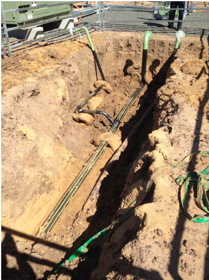
Plate 4-6 – HDPE gathering being connected to the well site
