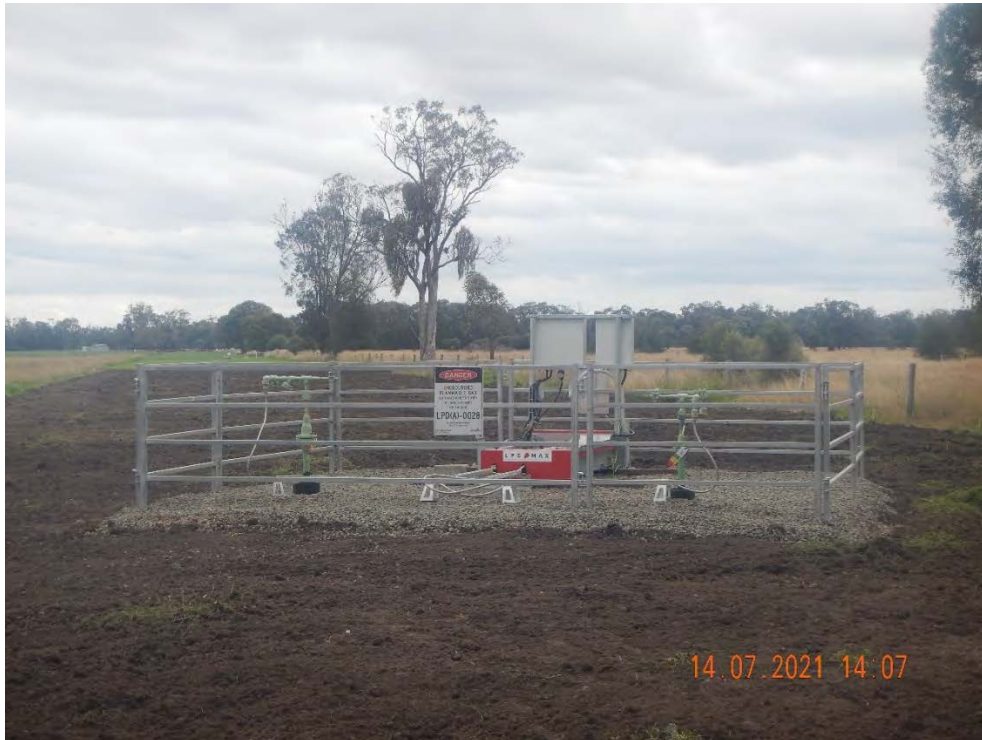
Plate 4-8 -- Image of a Low Point Drain
