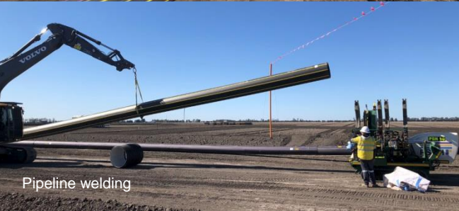
Stringing of pipeline ready for welding
