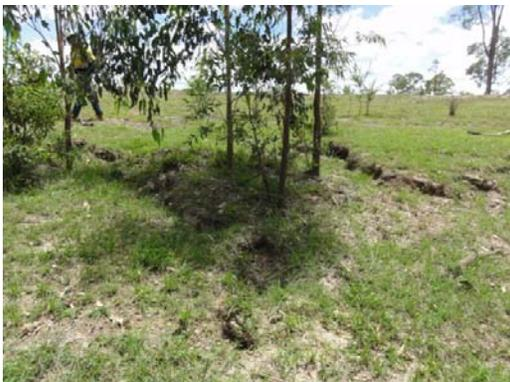
Tunnel erosion on the earthen bund built over the original wetland outflow point.
