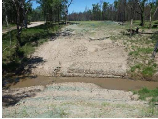
Origin Energy-Santos gas pipeline crossing on Dogwood Creek. Note the gully on the right bank (bottom left of photo) and the constriction of the channel.
