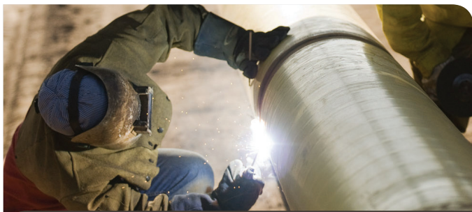
› Pipeline welding
