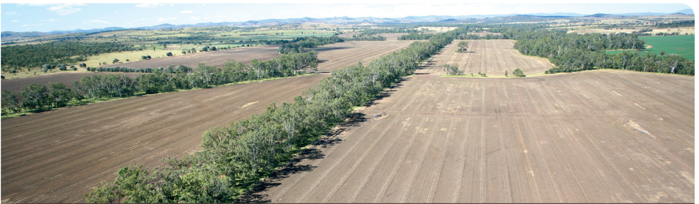
> Aerial view along the proposed pipeline route
