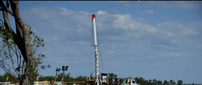
Construction of Plainview Pilot in 2018
