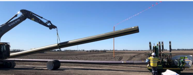
Pipeline welding at Plainview Pilot in 2018
