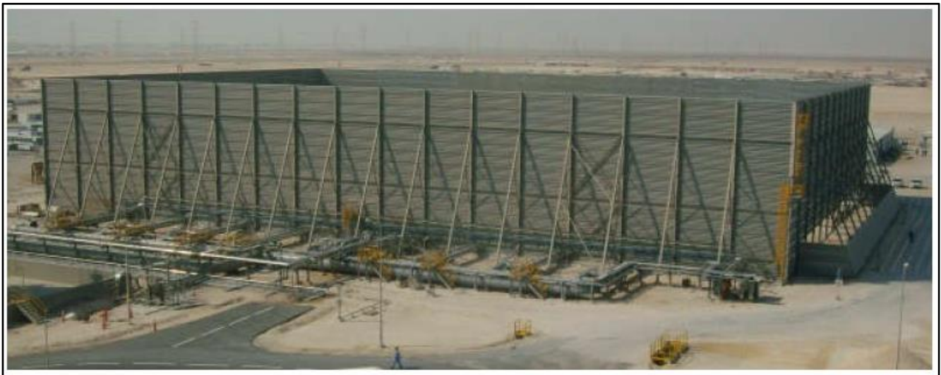
Figure 3 Indicative MPGF Fence (Image source: Zeeco)
