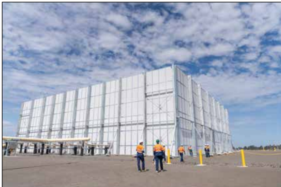
Figure 4-7 Indicative Multi-Point Ground Flare radiation fence
