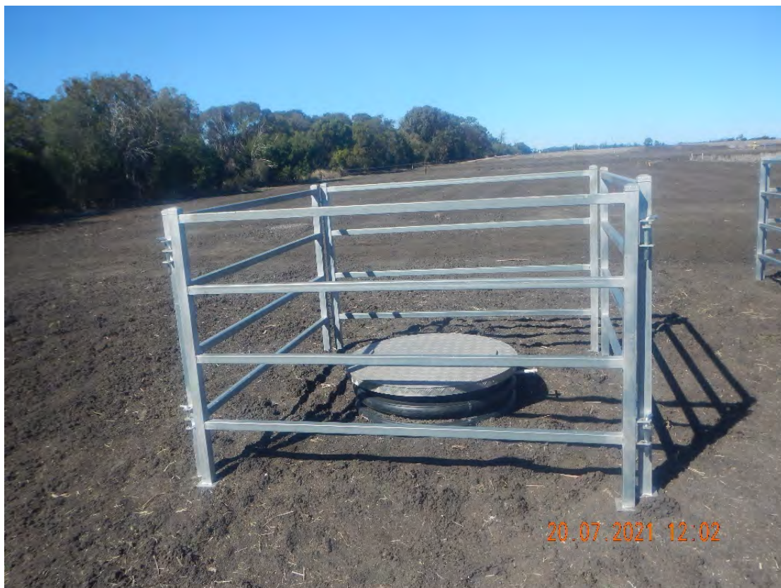
Plate 3-5 – Image of a valve post construction once the ROW has been backfilled
