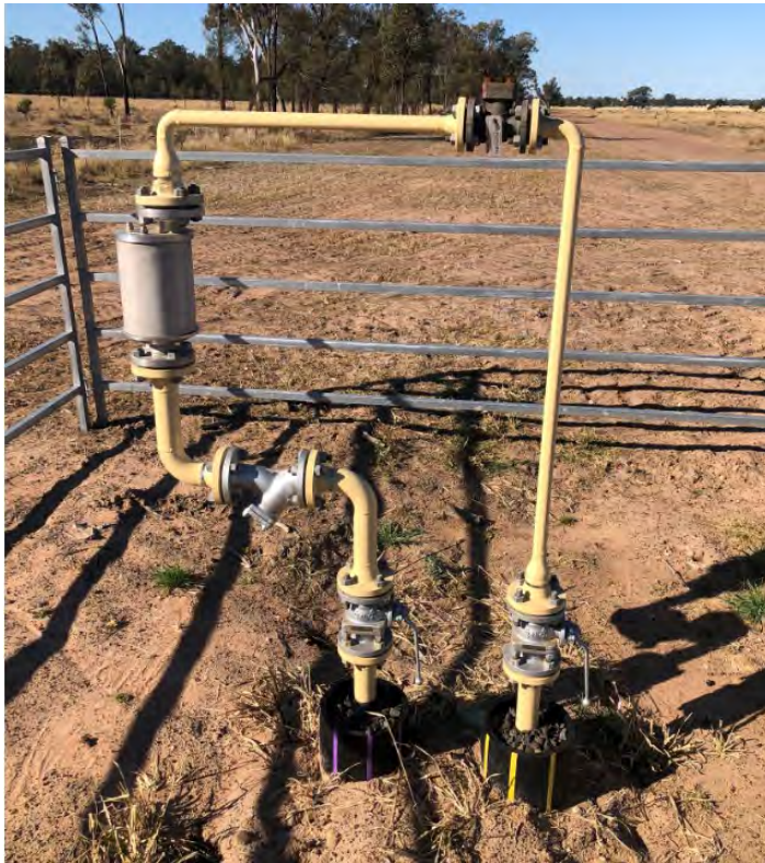
Plate 3-2 - Image of High Point Vent
