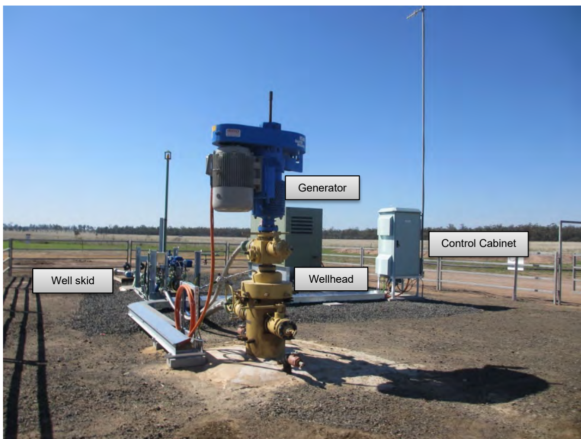
Plate 3-1 - Typical Well Head Facility and Infrastructure
