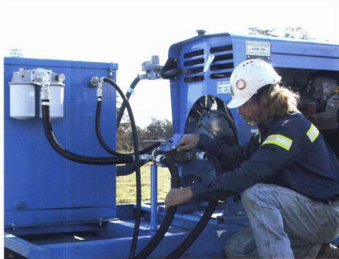
Mitchell Drilling undertaking well completion activity for Arrow Energy
